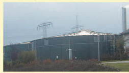
Biogas plant Rodewitz/Germany
