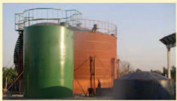
Demonstration project Cuba / Havana
