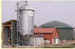
Biogas plant Dobberkau (Germany)
